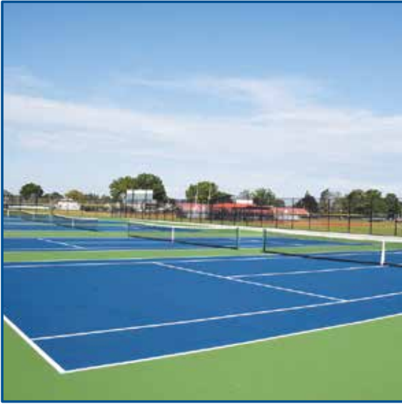
New tennis courts were installed at the high school.
